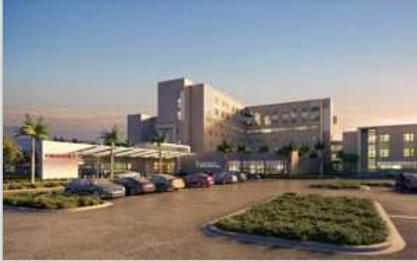
Skanska to Lead $229M Renovation, Expansion of Hospital in Southwest Florida
