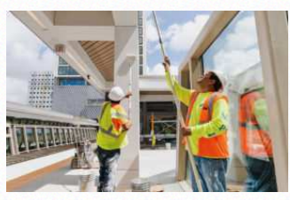
Photos: Finishing Touches At MiamiCentral Brightline Terminal
